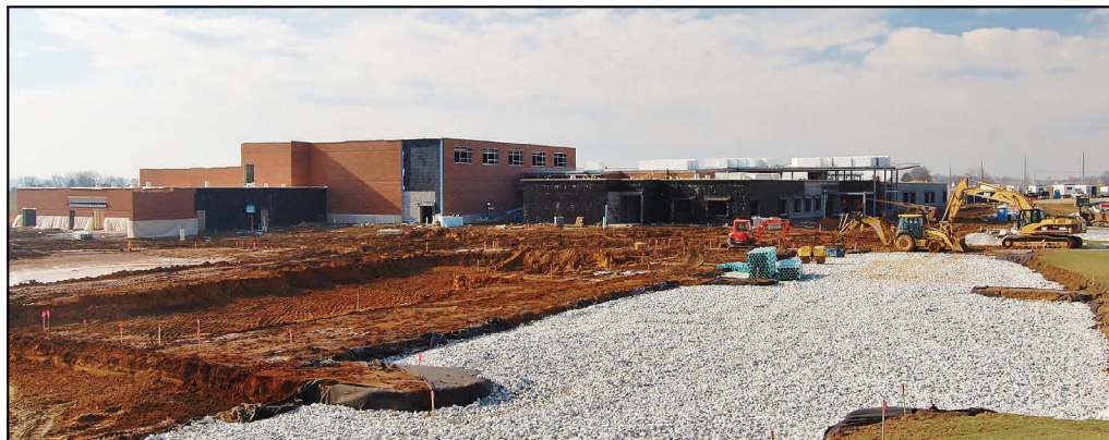
The new Hambright Elementary takes shape along Charlestown Road.
